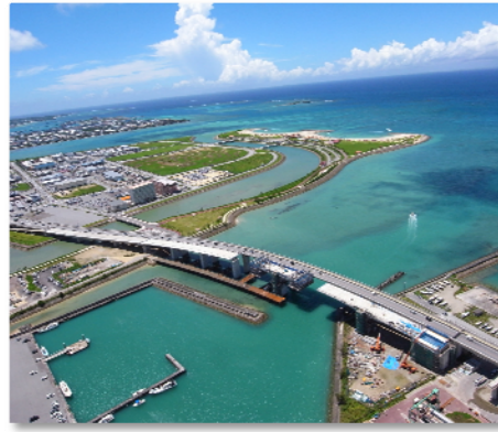
Tomigusuku Road Yone Bridge
