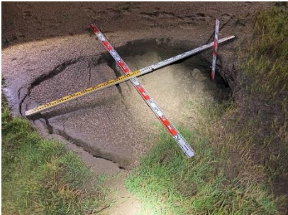
陥没 (1.8m × 1.4m × H0.7m)
