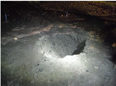
陥没 (1.4m × 1.1m × H0.9m)
