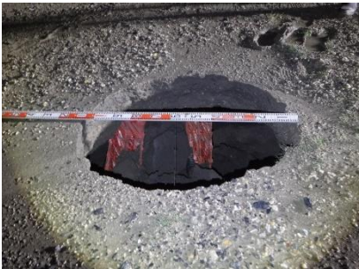
陥没 (1.1m × 0.9m × H1.3m)
