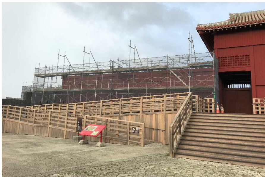
北側屋根を仮復旧中の奉神門
